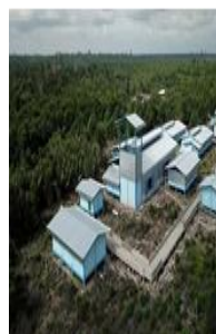
Figure 4. Integrated sago processing centre
